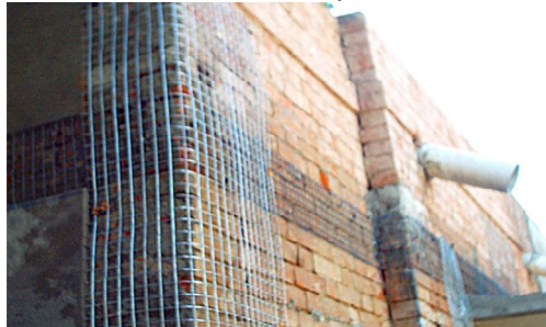
Figure 6: Seismic belt at outer corner
