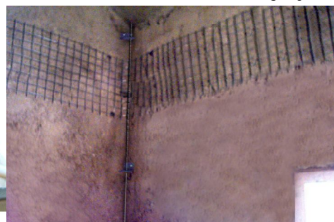
Figure 7: Inside corner reinforcement
