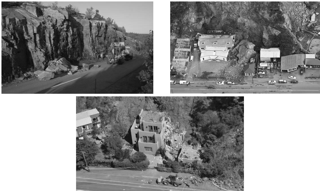
Figure 9. Some Examples of Structures Damaged by a Rock-Fall
