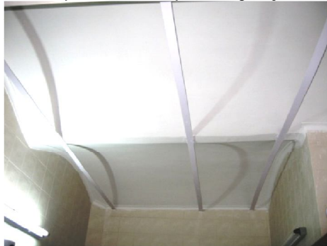
Figure 8: Ties in segmental arch construction
