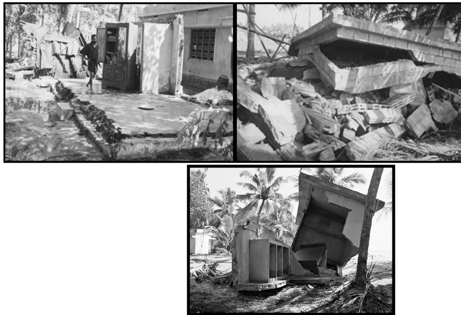
Fig.2 Pattern of Housing damages in Allapad Panchayath during Tsunami 2004 Strategy of Government for Rebuilding
