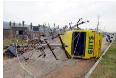
Power & Communication Failure poses major problem in post-cyclone scenario
